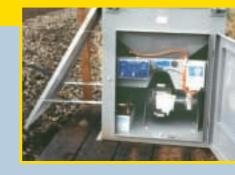
UK railways experience problems every Autumn when trackside trees shed their leaves. This installation uses a Watson-Marlow Bredel pump to feed gel-borne sand to the rails and increase grip for the trains
